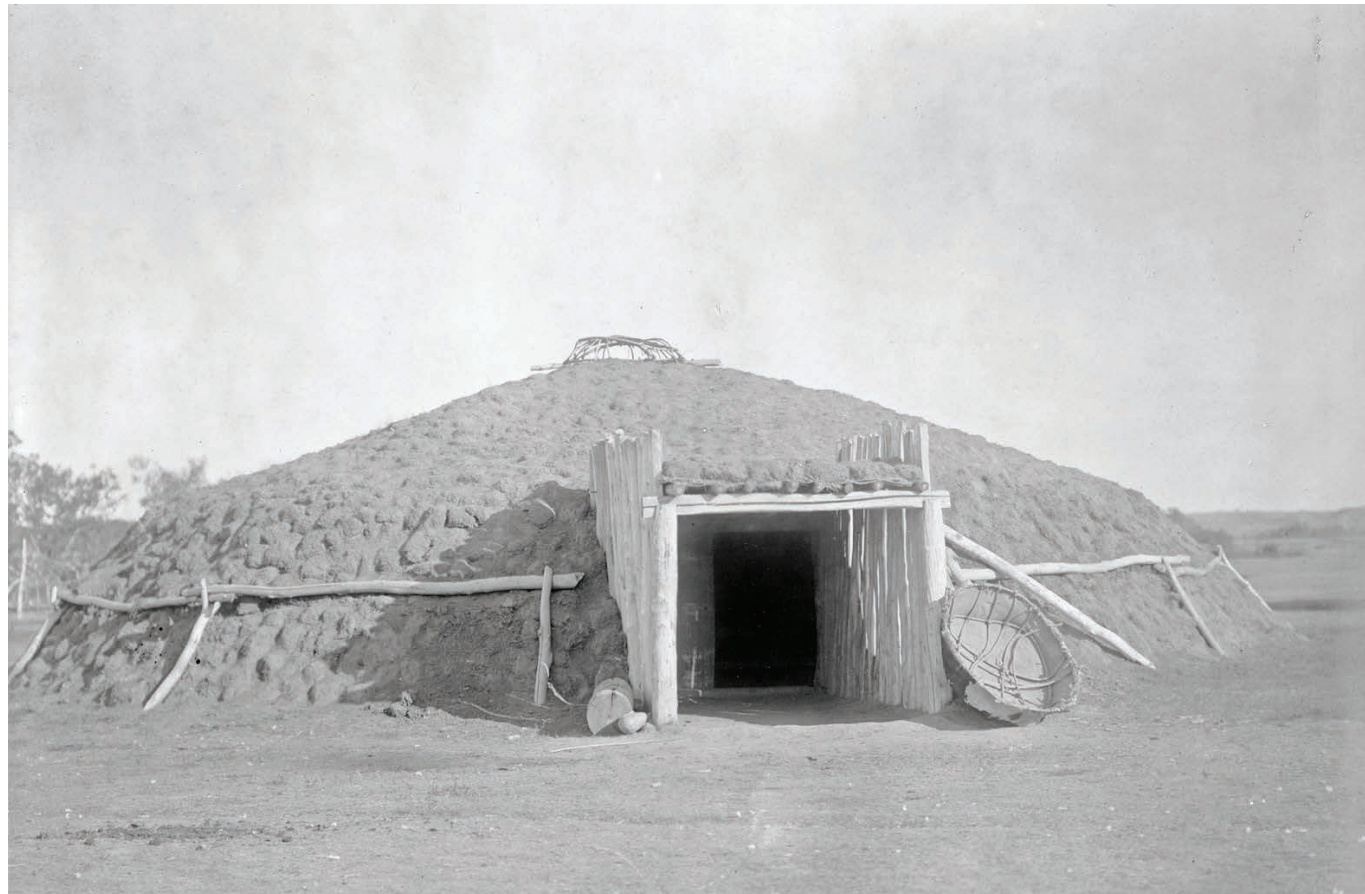
AN EXAMPLE OF A SKIDI LODGE FROM THE PAWNEE TRIBE OF NORTH AMERICA. AT THE TOP OF THE STRUCTURE IS A LARGE HOLE THAT WAS USED TO EXHAUST SMOKE FROM FIRE AND TO VIEW CERTAIN SECTIONS OF THE NIGHT SKY THAT WERE DEEMED IMPORTANT TO THEIR TRIBAL HIERARCHY AND TRADITIONS. IMAGE CREDIT: EDWARD S. CURTIS COLLECTION/LIBRARY OF CONGRESS, WASHINGTON, D.C.
